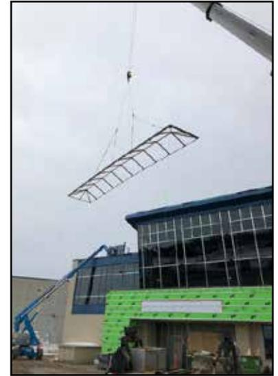
A crane lifts a skylight into place at Little Chute High School. Both paint and glass are working on this project.
