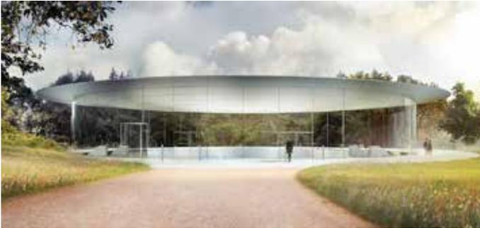
The thin roof disc comprises 44 identical radial panels, which are assembled on-site and carefully craned into position onto the completed glass cylinder in a single lift. All its services, such as electric conduits and sprinkler pipes, are invisibly integrated within the thin silicone joints between the curved glass panels.
